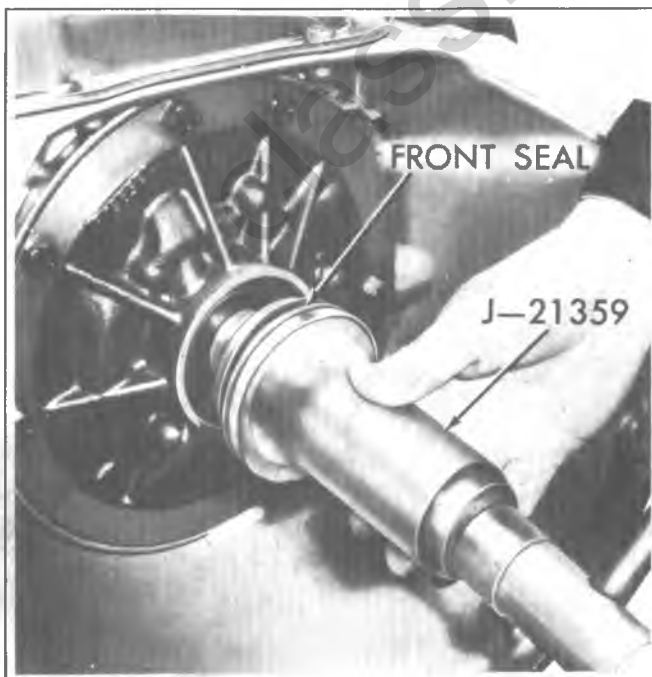
Fig. 7A-168C--Installing Pump Seal
