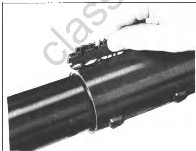
Fig. 3B4-29--Installing Switch Connector Onto Jacket Clips
