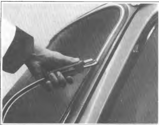
Fig. 2D-19--Installing Reveal Molding
