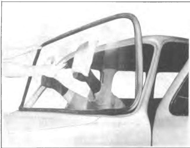
Fig. 2D-16--Removing Windshield from Opening
