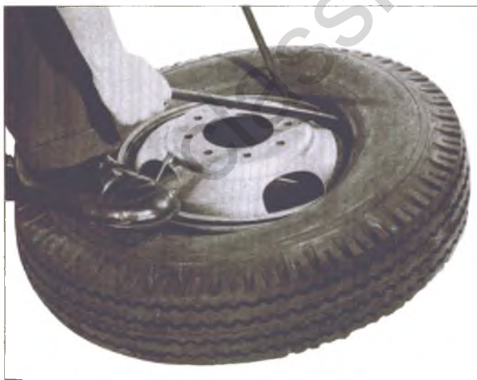
Fig. 8—Prying Bead Over Edge of Rim
