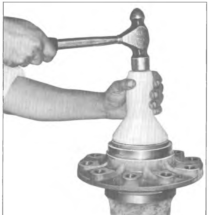
Fig. 76—Installing Hub Oil Seal
