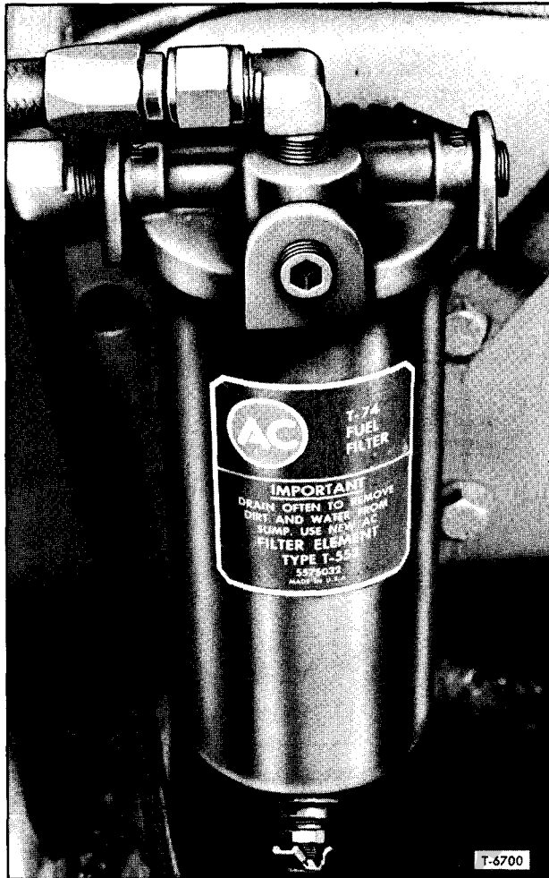
Figure 1—Primary Fuel Filter
