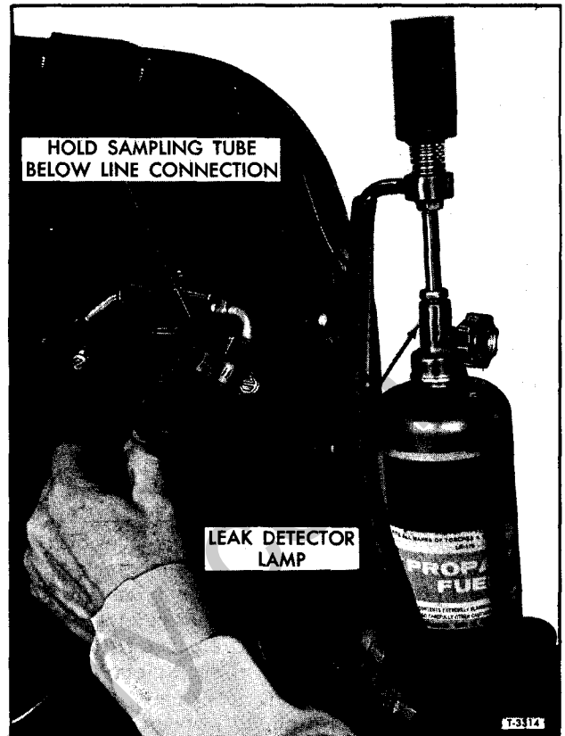
Figure 24—Checking for Refrigerant Leak
